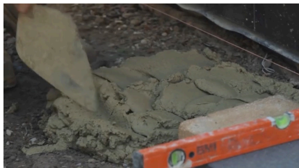
Spread thin layer of mortar for paver to bed on.
