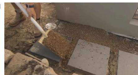
Spread pebbles in between paving slabs.
