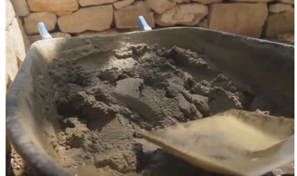
Mix mortar in a wheelbarrow using a 5:1 sand to cement mix.
